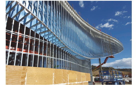
Exterior Framing for the Center
