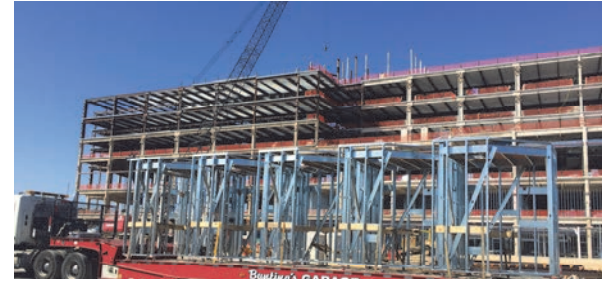
Pre-Fabricated Pods arriving at Bayhealth: Milford, DE
